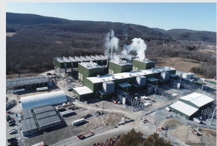
Cricket Valley Natural Gas Thermal Power Plant (generation capacity: 1,100 MW)
